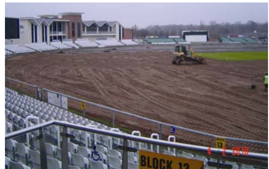
Root zone spreading Turf laying
