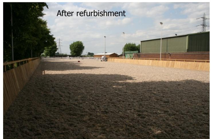
A bespoke fence was designed and installed, along with an extensive pipe drainage system to both arenas, installed using company owned laser guided machinery. Clean granite stone was imported to construct the arena base and high quality needle punched membranes, shipped from Belgium, were flame welded to encapsulate the drainage and stone layer.
